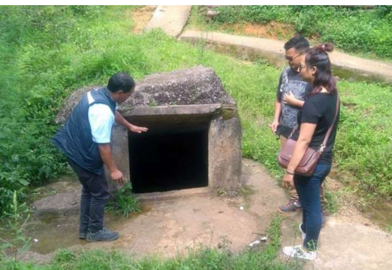
Figure 1. Mr. Bor Borshemlang Saiborne of NERCoRMP explaining how a spring tapped chamber has been constructed to tap the underground springs and help prevent sedimentation making it more hygienic for domestic use.
