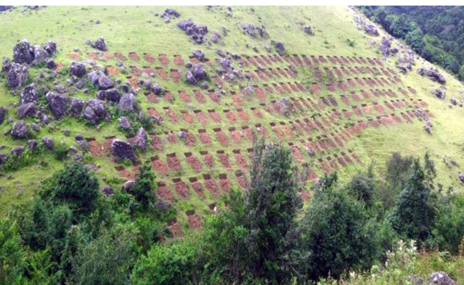
Figure 4. Staggered contoured trenches on the hill slopes of Mawthaidraishan, WKH to reduce run off and improve soil fertility.
